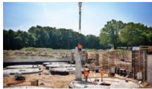
Picture gallery: Constructing a land-based salmon farm
